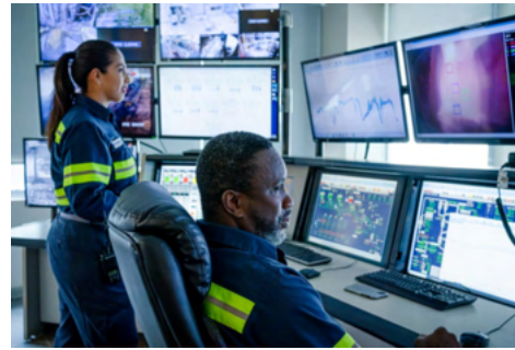
Control room at Pennsuco cement plant, USA.
