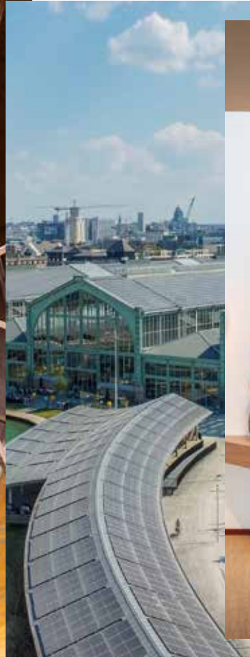
Nextensa > Solar panels for energy community
